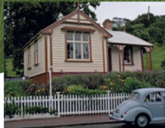
The Mangonui Courthouse was built of kauri in 1892. Until the 1920s, many houses were built from kauri. It was strong but light and didn't shrink or warp.
